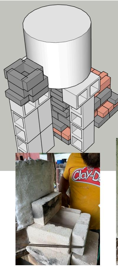
This layer of soft brick requires some notches to be cut and a brick shortened. Again, the hole should be about 7"x7". The chimney will sit on top of this layer. We added and 1' square of kaowool between this layer and the kiln to create a nice seal before adding the stove pipe.
