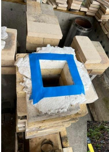
You can place tape upside down around the heat riser opening and set the kiln lid on it to determine where to cut. A cardboard template cut to  $\sim$ 7"x7" and set about 3" in from the edge of the bottom would also work. We cut the brick with a jigsaw and old blade after drilling holes in each corner.
