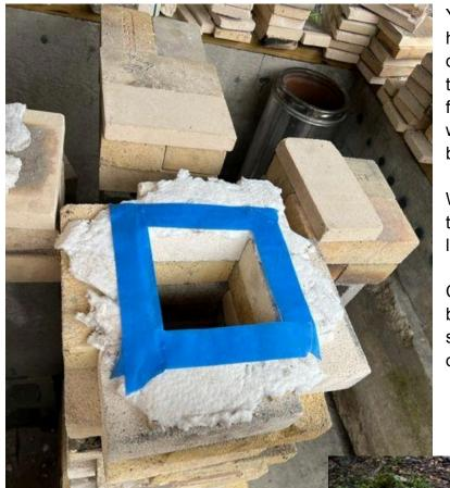
You can place tape upside down around the heat riser opening and set the kiln lid on it to determine where to cut. A cardboard template cut to ~7"x7" and set about 3" in from the edge of the bottom would also work. We cut the brick with a jigsaw and old blade after drilling holes in each corner.
